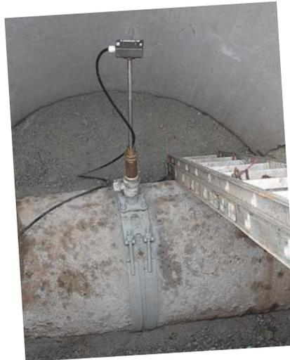
Failed in-line meters can even be left in place, as long as they do not interfere with normal pipeline operation. This eliminates expensive bypass and re-routing costs.
