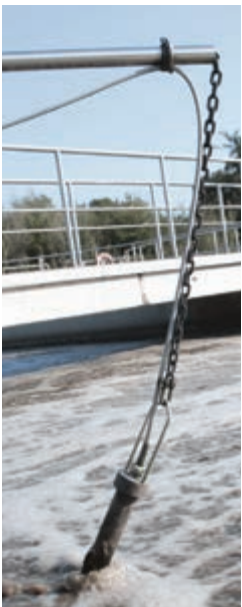
Chain Mount Provides self cleaning, shown with single sensor holder
