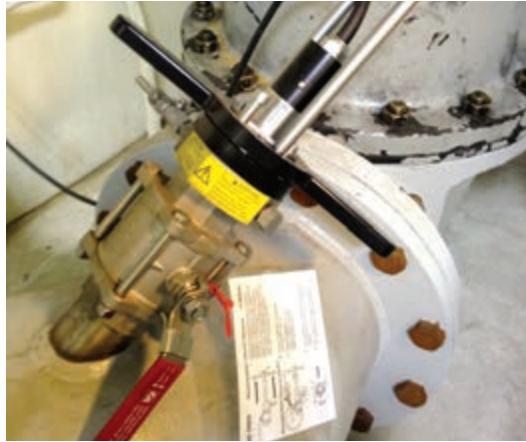
Pressurized, retractable insertion mount 2 bar or 10 bar overpressure
